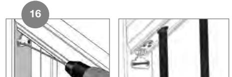
Secure the top rail to the post at both ends using the supplied 2 in. screws. Do not over tighten.
