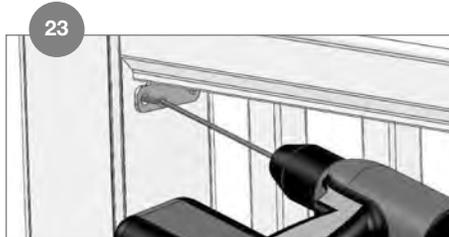
Secure the top bracket and rail to the post using the supplied 2 in. screws. Do not over tighten.
